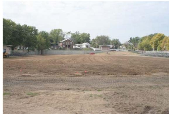
2. Start by measuring and marking out the entire area to be sodded. Use marking flags for the corners, and lay a string line down the center along both axes.
