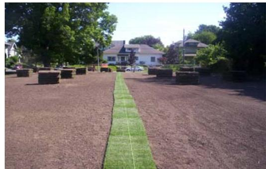
2. You will be working outwards from the center line towards the edges. The sod pieces should rest as closely as they can to one another, and should be placed in single columns as the volunteers work their way across the area. Once a column is complete, go back to the top and continue working your way back down. Divide up your team into loaders, carriers, placers, and quality control. Please handle the sod gently. It is a living plant and can die... and we do not want that to happen!
